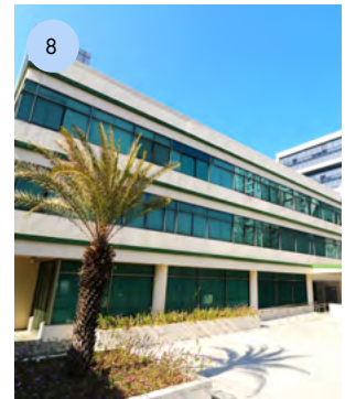
Plaza A Grade A, PEZA-accredited Year Completed: October 2007 GLA: 10,860 sq. meters
